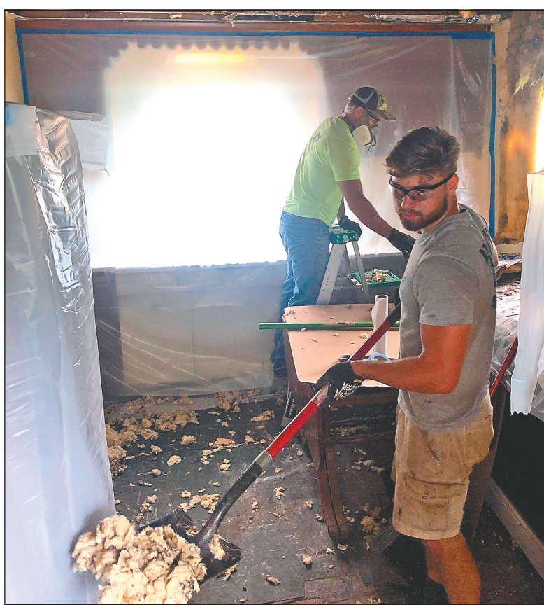
A Dreamers crew works inside one of the residential buildings.
